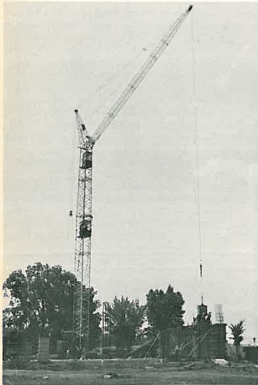
Construction on the new building off the New Benton Highway is coming right along, as you can see. The huge crane being used is as tall or taller than the 10 floors which the new structure will have. In the picture at left, concrete is being poured for the west wall. Above is the east wall. The crane rolls along on tracks like a railroad, and is used to lift sections of walls in place.
